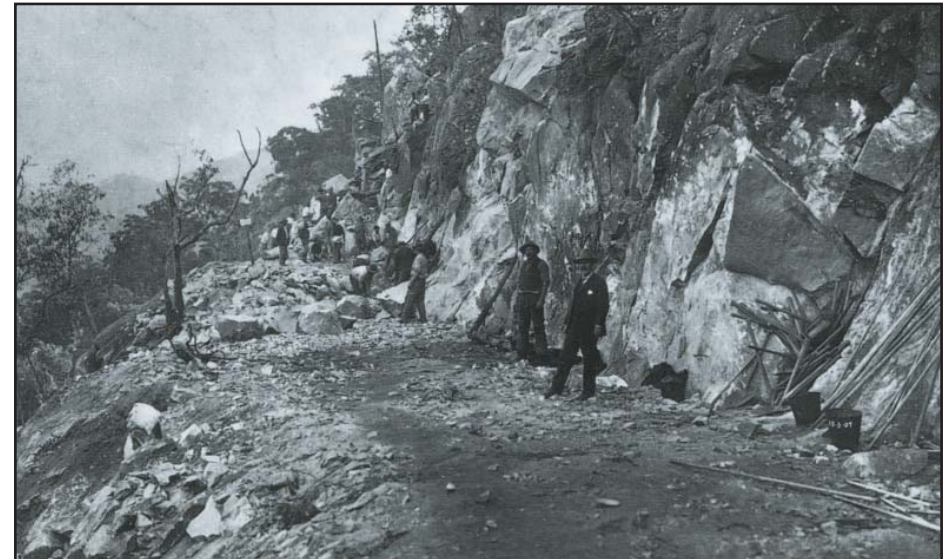
Barren Jack (Burrinjuck) - 15 May 1907. Labourers working on the construction of the railway along Carroll's Creek.
